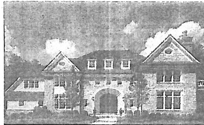
This property designed by R. S. Granoff Architects was named 'Best Spec Home: $5 - $6 Million.'
